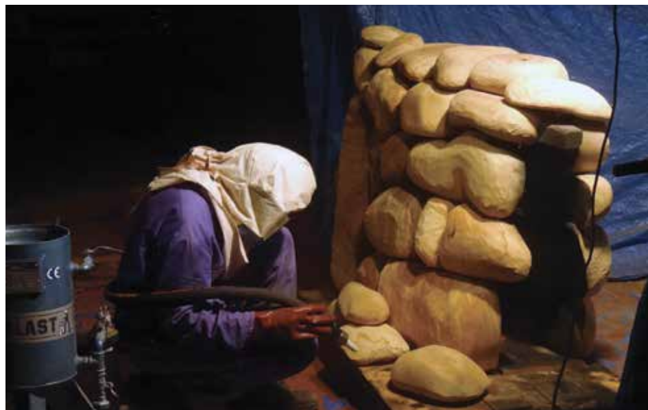
John sandblasts the wall, late at night.
