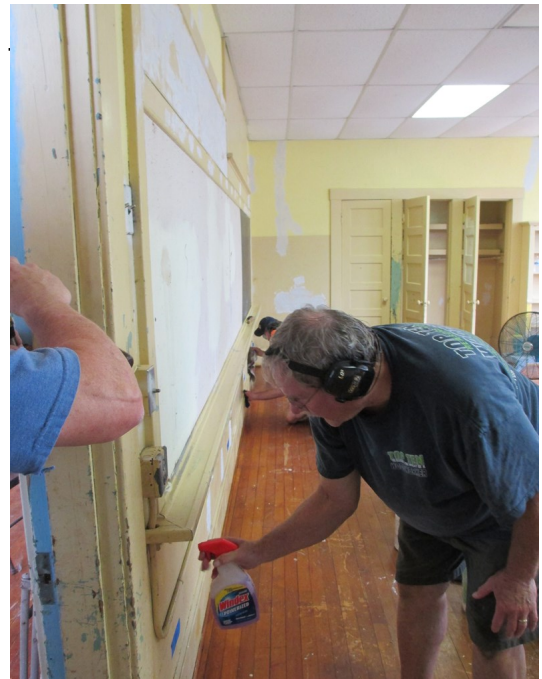
Dennis Hippen at work scraping paint
