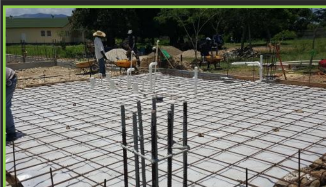
Installed plumbing rough in and poured slab.
