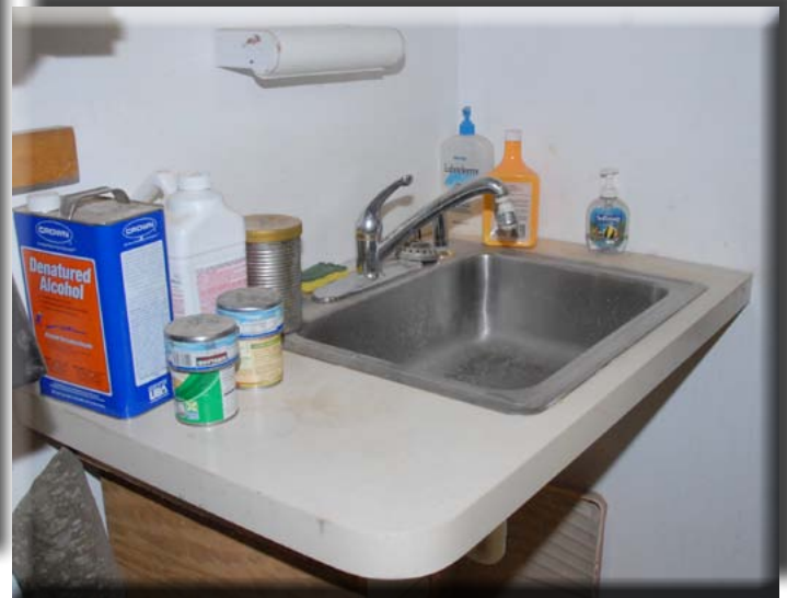
Often overlooked when designing and building a shop, a sink is a valuable addition. Adding one required that Tom hammer-drill his way through the concrete basement floor, patch into the drain, and run hot & cold water through the wall near his furnace. The next best would be a partial bath room, or even a full bath that would permit comfortable living when installed in the "husband" dog house. We have all been there.
