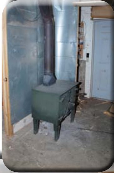
The heat source is fed by scraps, and wood that was left unattended too long. Note the system of heat protecting panels.
